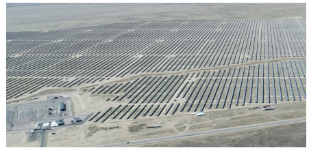
The overview of Kapchagay 100MW Solar Power Plant
