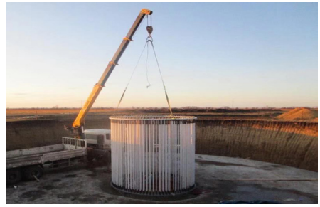
Anchor Bolts have been installed for the first wind turbine foundation
