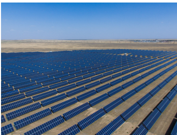
Zhanggiztobe 30MWp Solar Power Plant
