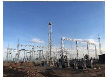
Kapshagay 220kV Substation
