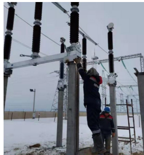
Installation of disconnectors
