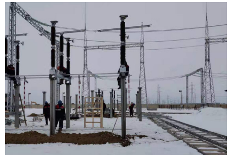
the newly added bay of connecting point for 220kV side
