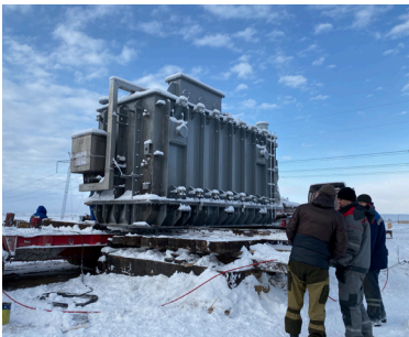
The Power Transformer at the project site
