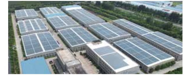
Industrial and Commercial Photovoltaic Power Station 5.99 MWp Roof-distributed Photovoltaic Power Station in Zhejiang Province
