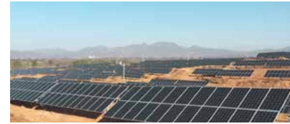
Ground-mounted Photovoltaic Power Station 35 MWp Photovoltaic Power Station in Hebei Province
