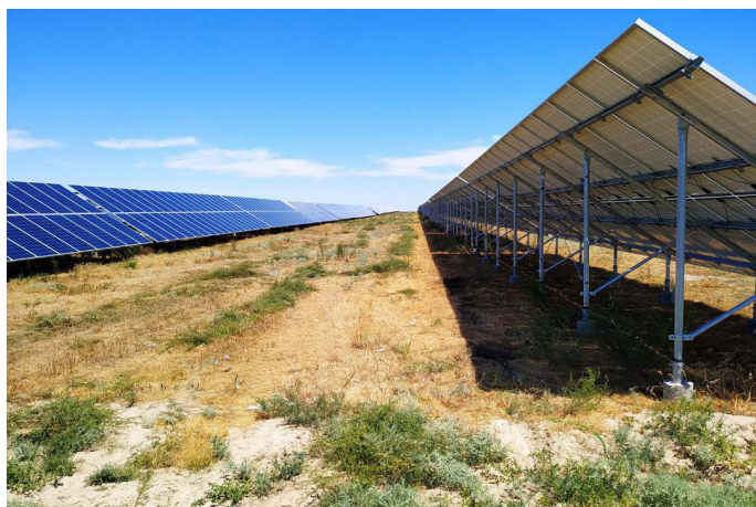
▲ 三等奖：Zhangiz 30MWp 光伏电站风貌 / Nurzhan Jakanov
