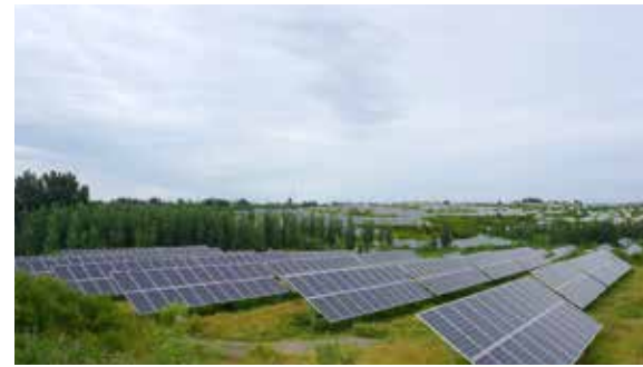
Centralized Ground-mounted Solar Power Plant
