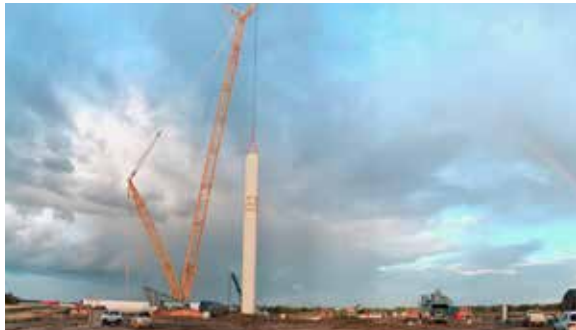
Wind Power Plant in Plain Areas
