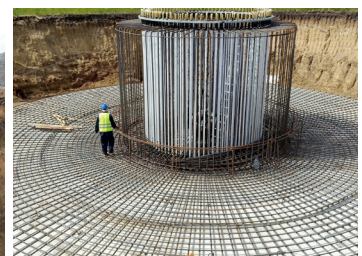
The foundation construction of the project
