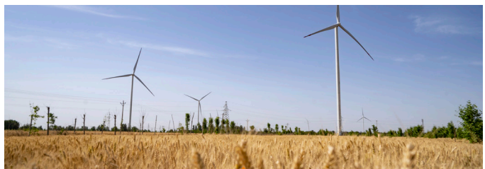
▲ Baixiang 50MW Wind Power Project
