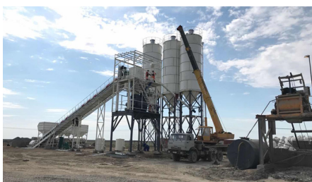
The concrete mixing station of Abay 100MW+50MW Wind Power Project
