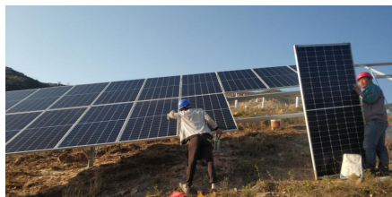
UNIBLU team is working hard installing PV panels
