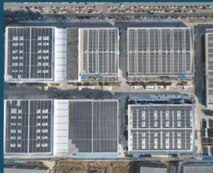
Tianjin 5.07MWp Distributed Solar Power Plant
