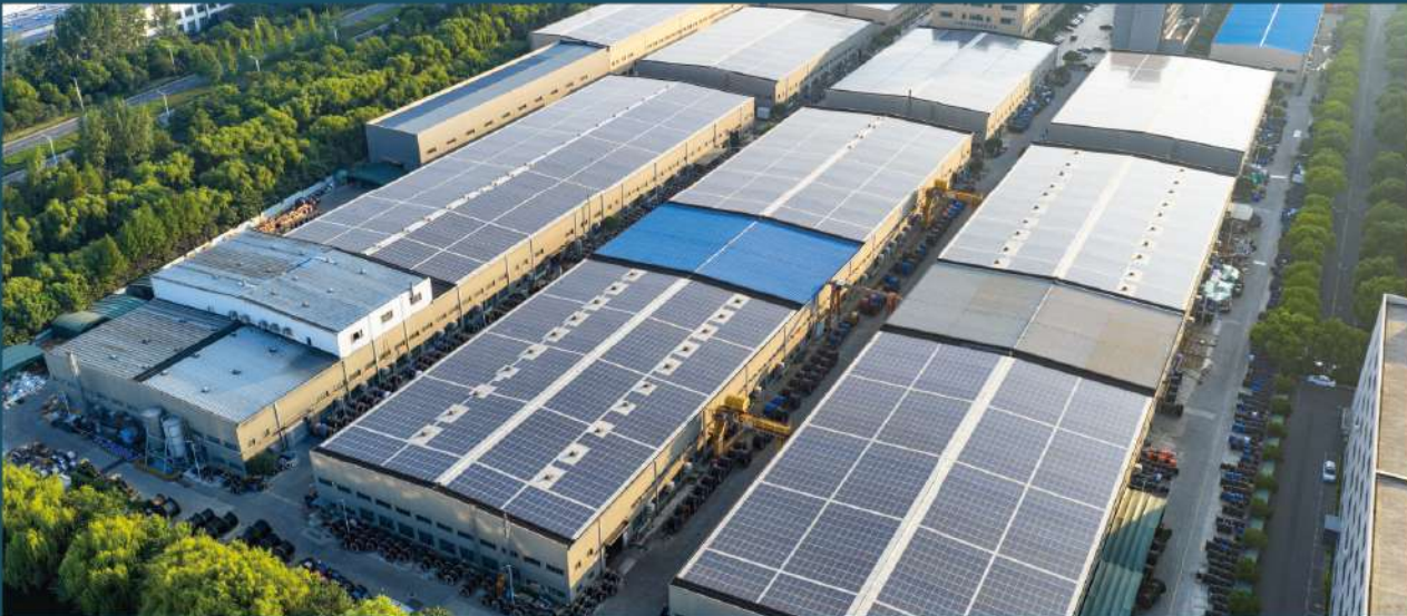
Hangzhou 5.992MWp Distributed Solar Power Plant
