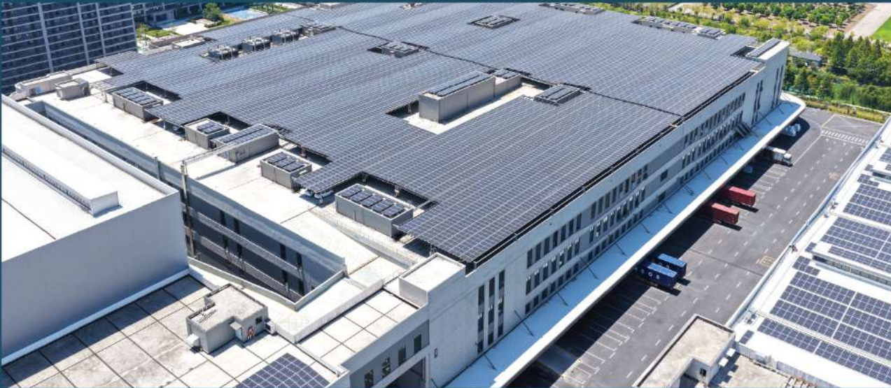
Hangzhou 12MWp Distributed Solar Power Plant
