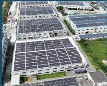
Taizhou 4.91MWp Distributed Solar Power Plant
