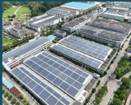
Taizhou 3.188MWp Distributed Solar Power Plant
