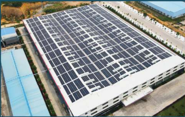
Guangxi 1.94MWp Distributed Solar Power Plant
