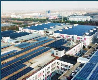
Hangzhou 5.7474MWp Distributed Solar Power Plant
