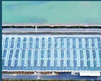
Shaoxing 6MWp Distributed Solar Power Plant
