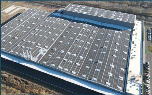
Tianjin 6MWp Distributed Solar Power Plant
