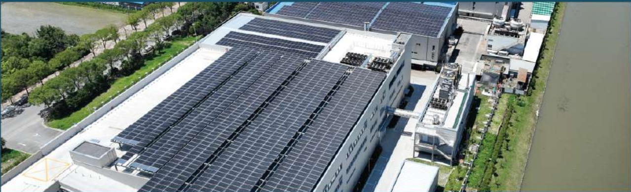
Shanghai 2.1MWp Distributed Solar Power Plant
