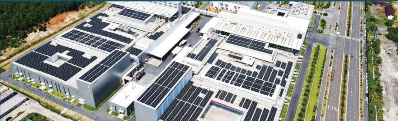
Jiangxi 4.88MWp Distributed Solar Power Plant
